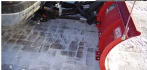
One-quarter-inch aggregate is swept into paver joints.
