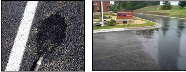
Close up of water pouring onto porous asphalt. Porous asphalt on the left, traditional street on the right. Both photos courtesy of Ramsey-Washington Metro Watershed District.
